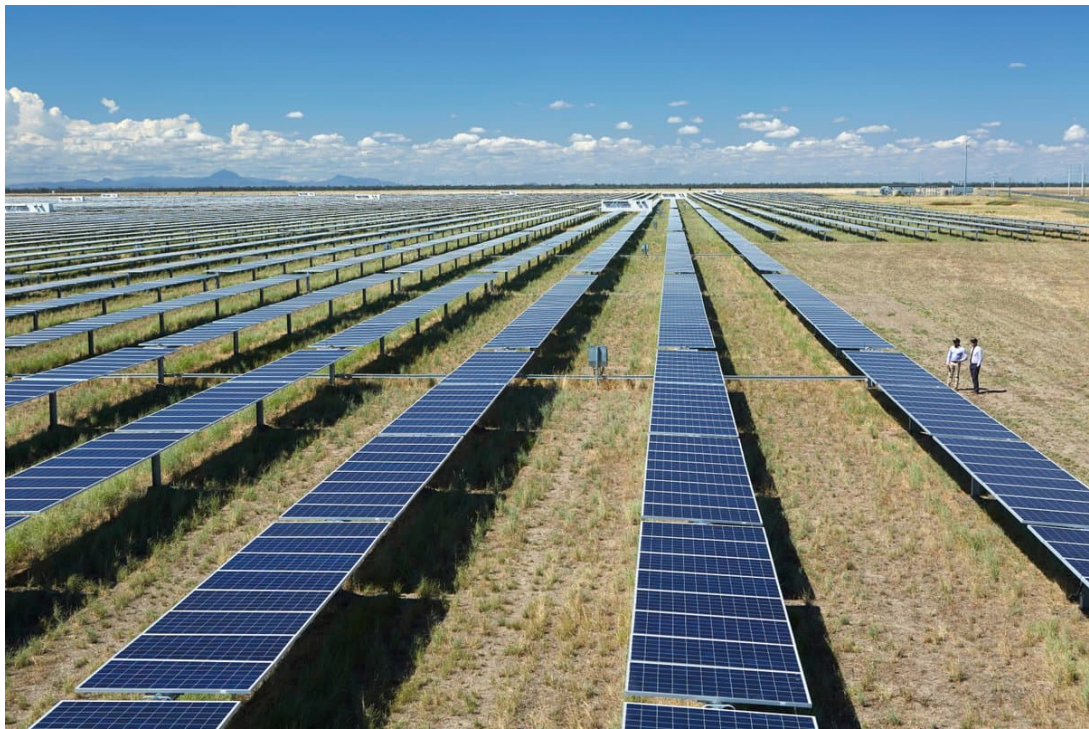
Plate 3-2: Single-axis Tracker Arrays
